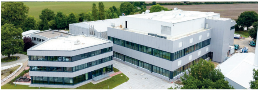
Richter-Helm's expanded manufacturing site at Bovenau, Germany – ready to manufacture your product
